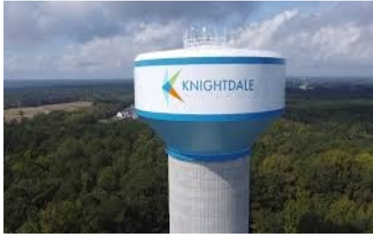
Hodge Road water tower
